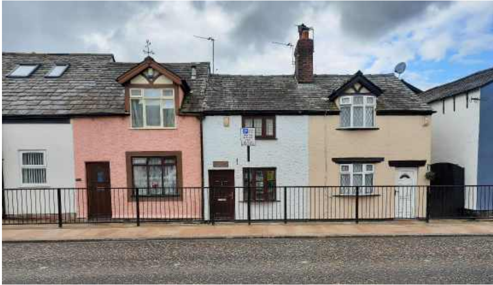
Garstang Road 18 th Century Cottages
