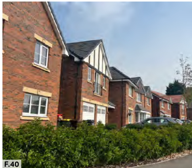
Figure 40: Stewart Milne Homes - Broughton Park development
